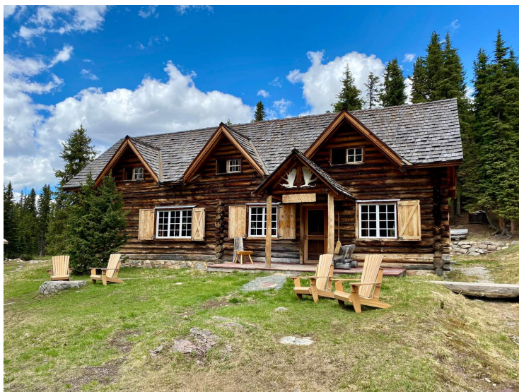
Figure 2: Skoki Lodge log buildings in a grassy backcountry clearing.
